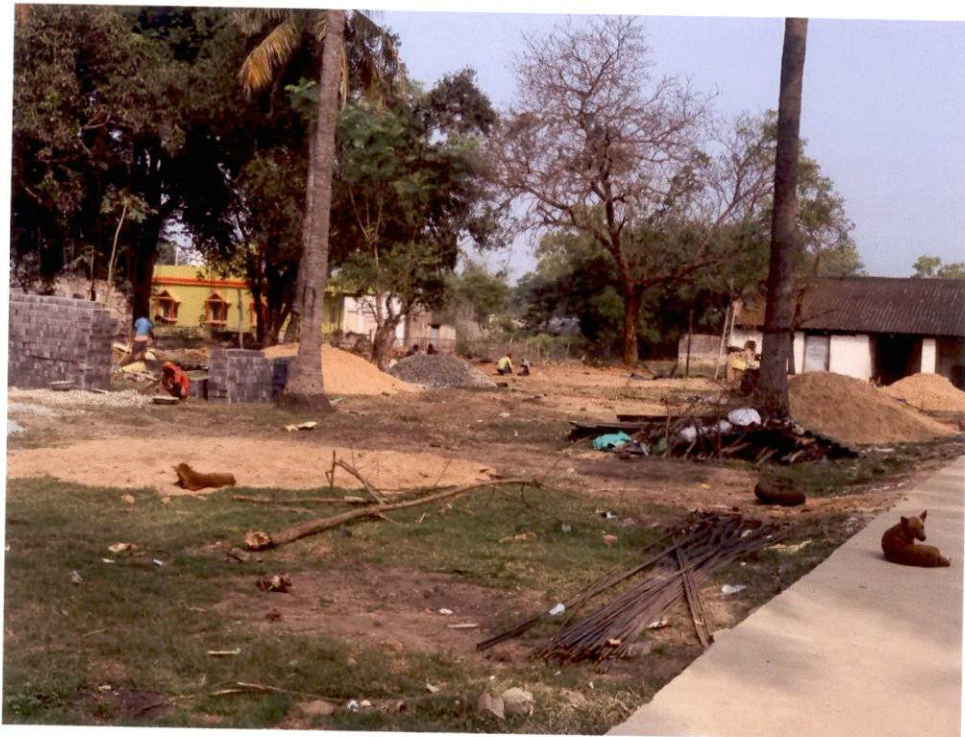
2. HOUSES UNDER CONSTRUCTION: OCCUPANTS ADJUSTING ELSEWHERE
