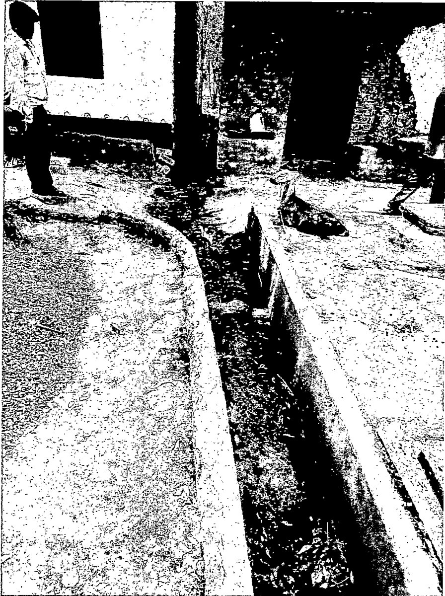
Photo of Open Drain
